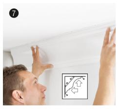
**Push firmly** I Ensure that you apply the marked edge to the ceiling. Put the crown molding into place, checking that it is horizontal and symmetrical to the wall and ceiling. When you are confident the molding is positioned correctly, firmly press it to the wall and ceiling across the entire length.
