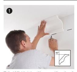
**Mark out** | Mark the bottom of the crown molding on the wall. Make sure the molding is positioned correctly at 90°.
