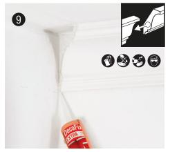
**Use DecoFix Extra on every joint** I Butter up each end with a complete covering of DecoFix Extra adhesive. Read safety instructions on cartridge.
