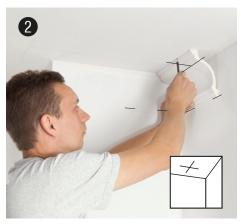
**Draw the miter angle on the coving** I to make sure you place the frame correctly in the miter box.
