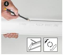
Marking the ceiling side | Add a black line to the ceiling side of the coving. When cutting, place black line edge at bottom of mitre box! With other words, flip the molding.
