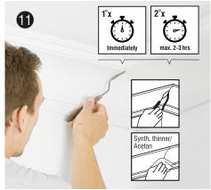
**Clean** I Wipe off the residue immediately so that it is flush with the molding. You can repeat this process one hour later. Use a cloth dipped in pure acetone to remove adhesive residue.
