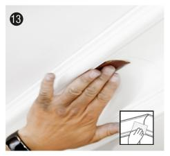
**Prepare for paint** | All Orac Decor® moldings are pre-primed in white, but still need to be painted over with a suitable paint. For good adhesion, lightly rub the length of the moldings with a 320 gram sandpaper.
