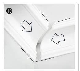
**Push** both moldings firmly and securely together. Excess adhesive should seap through the join.
