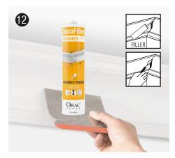
Use DecoFiller to smooth out all visible joints | If there are minor irregularities on your molding and/or wall joints these can be filled with our FL300. You might find it easier to do this 24 hours after the initial installation.
