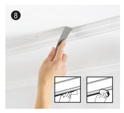
**Cleaning overspill** | Any overspill of DecoFix Pro can easily be removed with water. Any overspill of DecoFix Power can easily be removed with water and soap.
