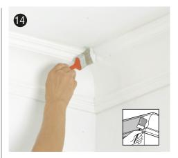
**Decorating** I Allow at least 24 hours before decorating your Orac Decor® products. For best results add an undercoat and top coat of paint. On new builds apply a mist coat and top coat the following day.
