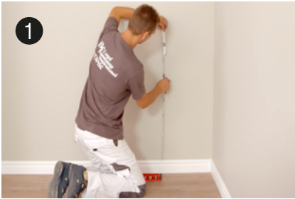
1 Measure | Measure the distances to wall/floor required.
